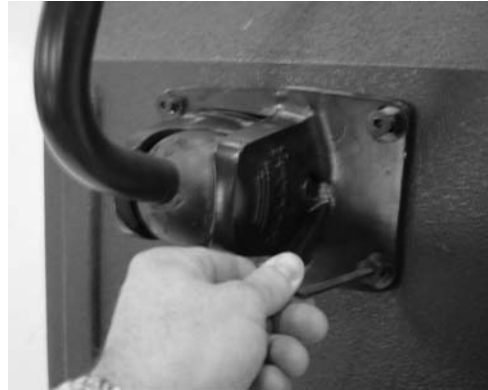
(2) Attach Omnimount plate to enclosure
